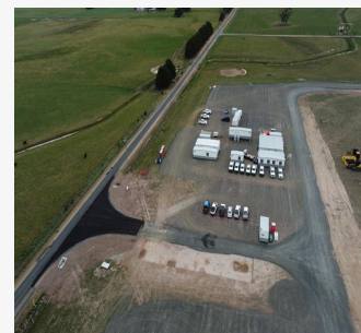
Main contractor compound.
