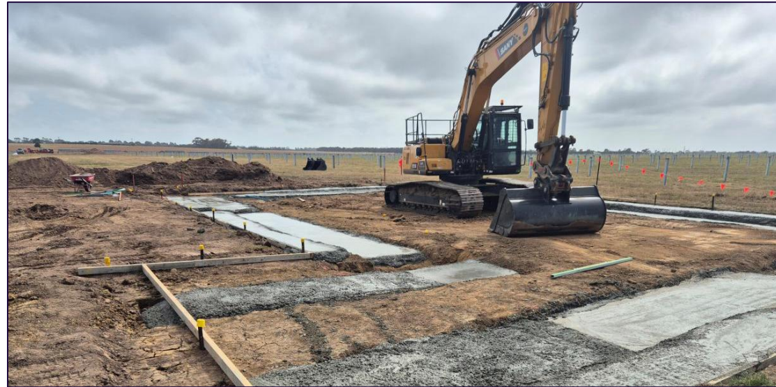
Figure 16: BESS bund construction
