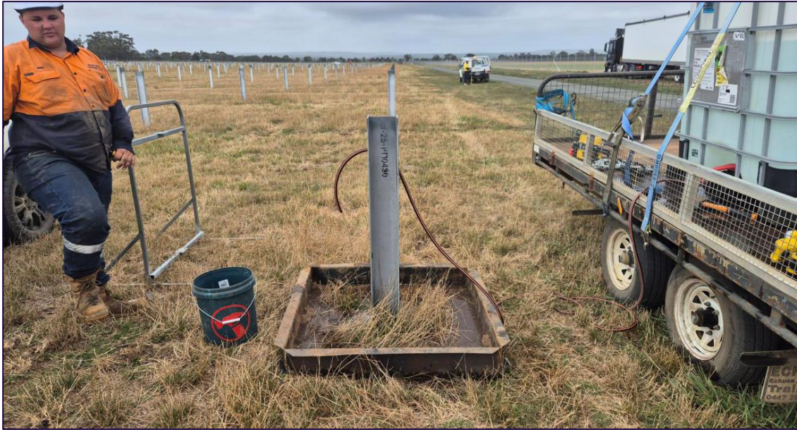
Figure 13: Tracker pile – pull out testing
