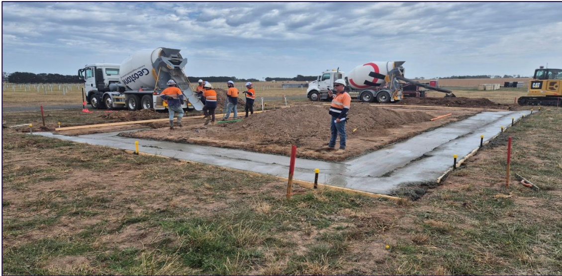
Figure 11: BESS bund construction, concrete pour
