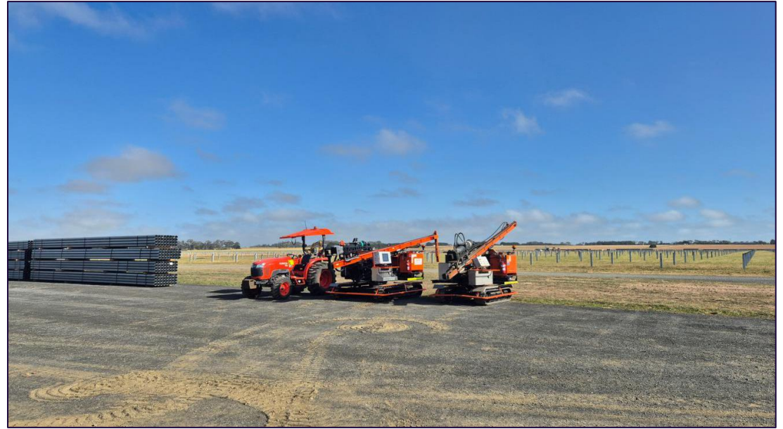
Figure 10: Additional piling rigs mobilised at site
