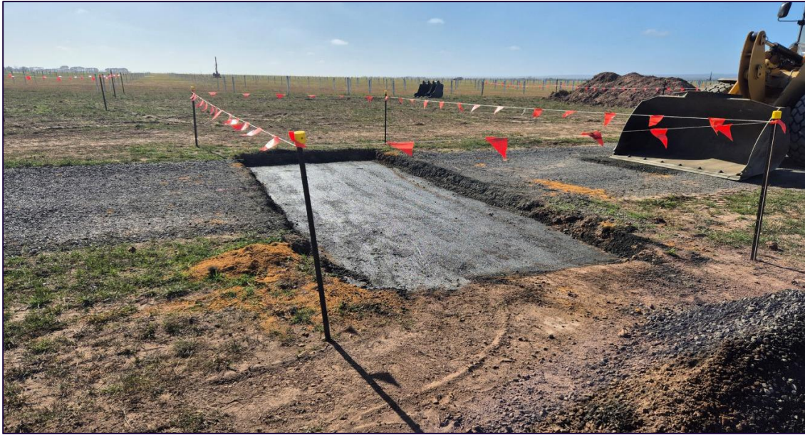
Figure 9: Back filling of road crossing trenches
