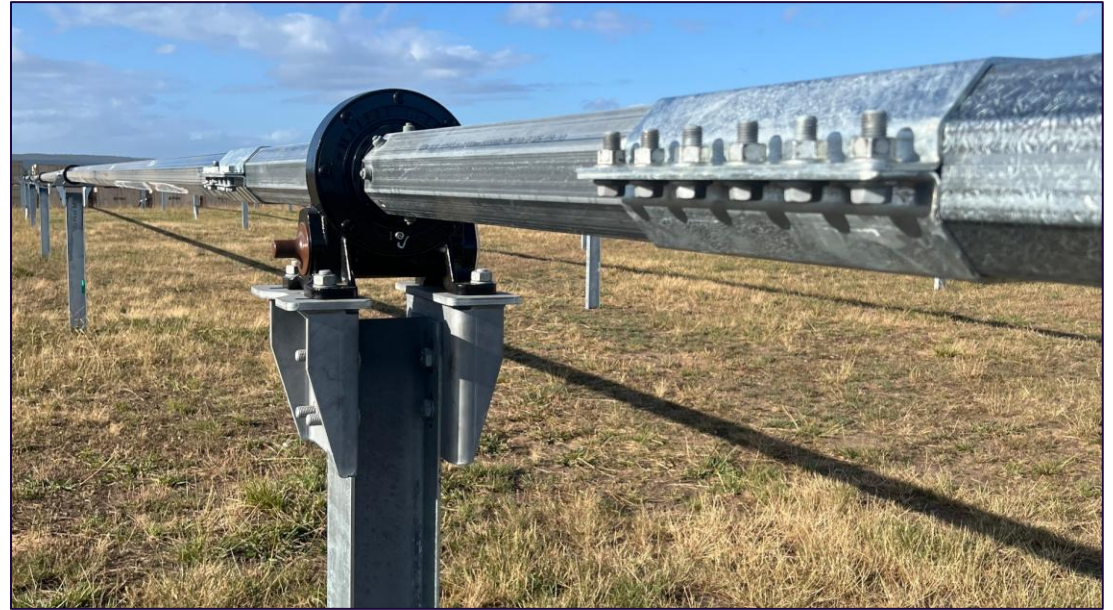
Figure 6: Tracker row installation
